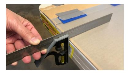
To mark a line parallel to the "clean" lengthwise edge, use a right angle to place guide points exactly 5 in (12.7 cm) into the acrylic sheet. A crooked line will yield a sidewall of uneven height.
